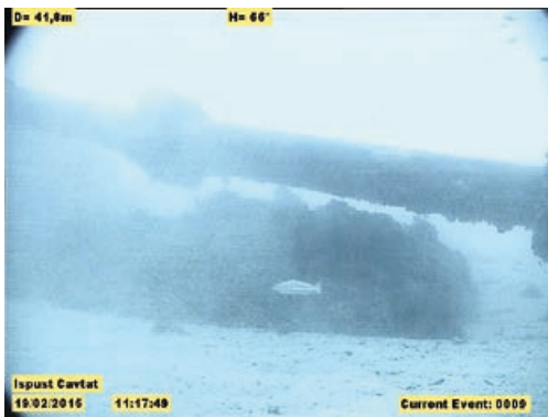
Outfall in Cavtat in Croatia
